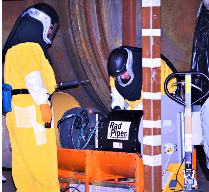
Fig. 1. Technicians prepare to deploy PCAMS RadPiper into a contaminated process pipe.
