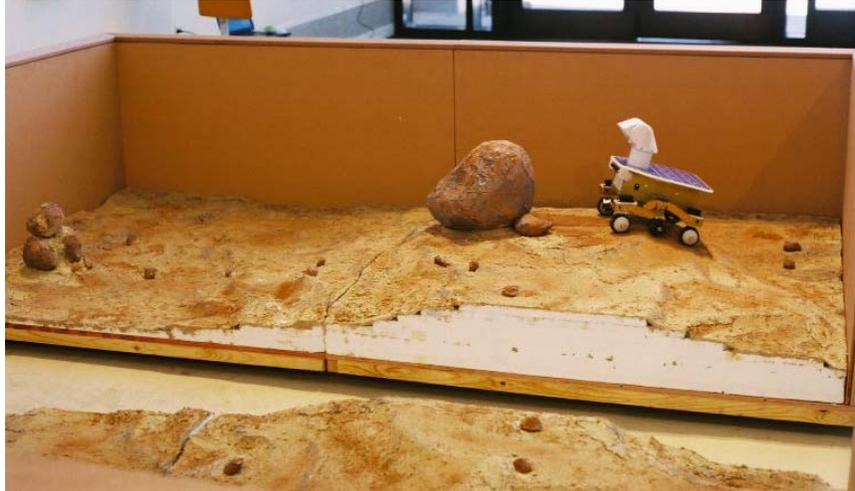
Fig. 9. This picture of the Smithsonian Air and Space Museum yard was taken during installation of the exhibit, before the horizon images were added. The yard is built on casters and designed to split into four quarters so that it can be easily moved.
