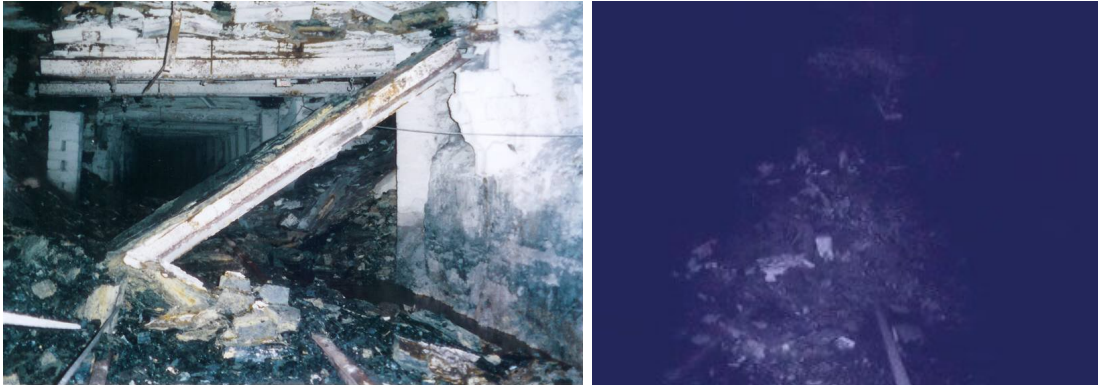
Figure 6.16: Obstacles encountered by Groundhog during the exploration of the Mathies abandoned mine. Fallen roof beam (left) and complete roof collapse (right)
