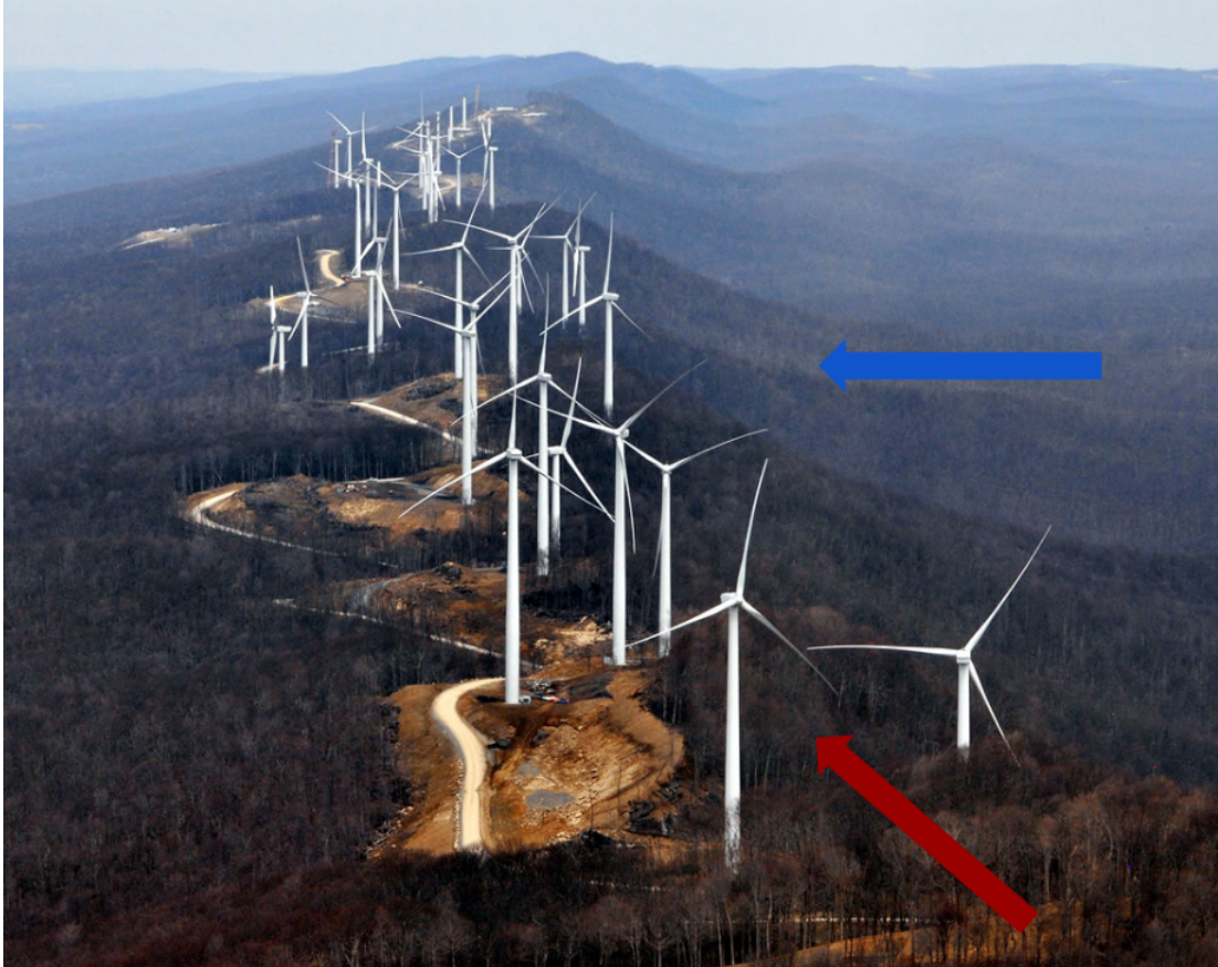
Figure 1.1: Laurel Mountain Wind Farm in West Virginia. If the wind flows over the ridge (the blue arrow in the image), then the turbines will yaw to align with the wind to generate maximum power. If instead the wind flows along the ridge (the red arrow in the image), then yawing to align with the wind causes the turbines to form a column, resulting in wake interactions that reduce power greatly. Source: John Terry
