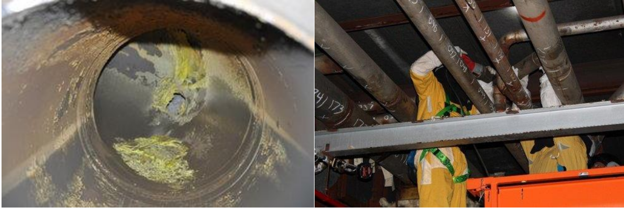
Figure 1: Leftover deposit in 42" piping (left). Manual inspection of small piping (right).
