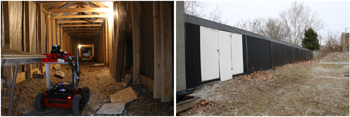
(a) Robot Inside of Tunnel
