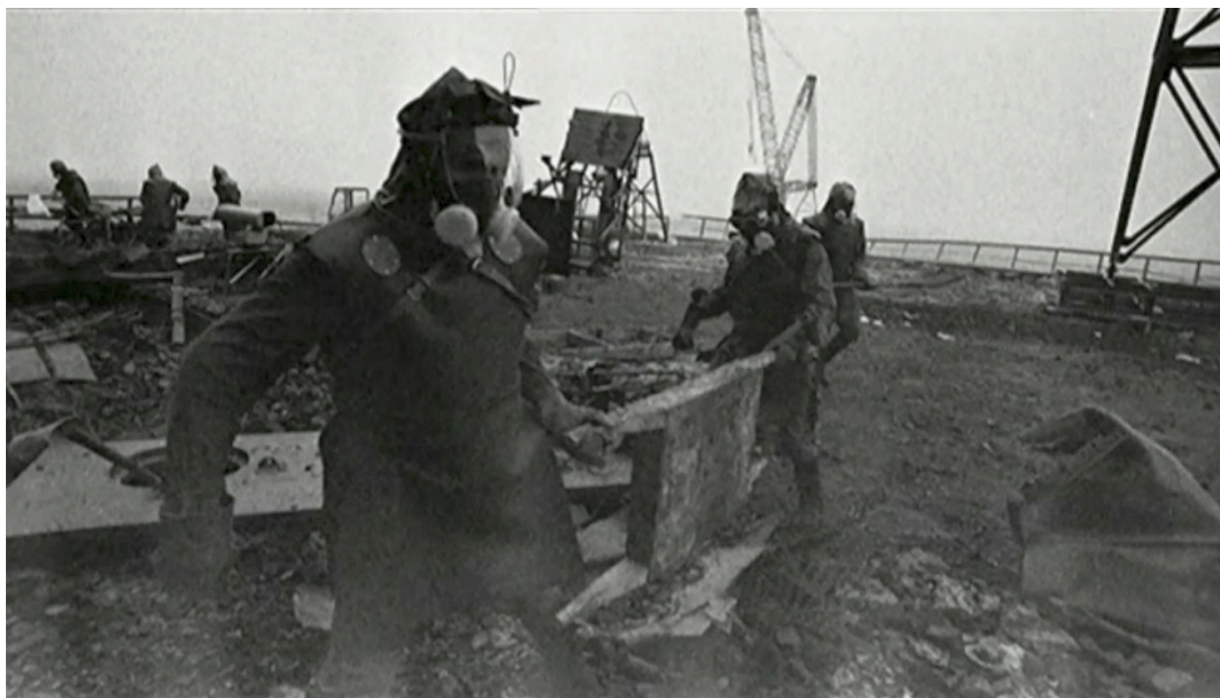
Figure 1.1: Workers removing radioactive graphite at the Chernobyl nuclear facility in 1986
