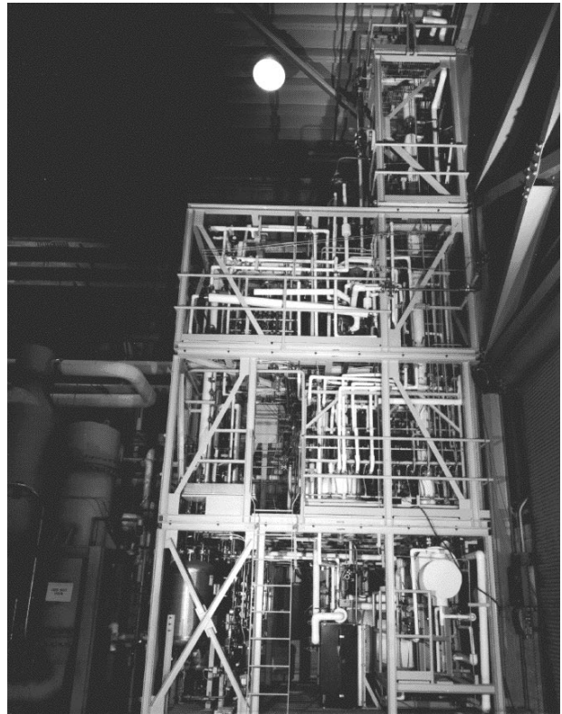
Figure 1. The IODOX facility, a DOE test site for selective equipment removal.
