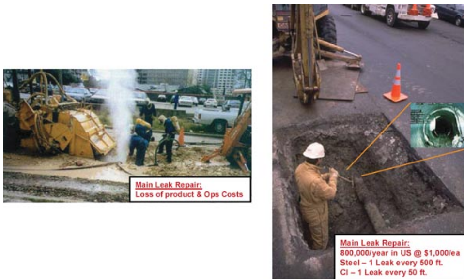
Figure 1. Currently employed leak-search and repair process.
