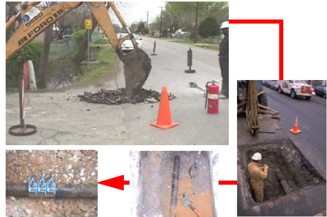
Figure 3 : Conventional leak-repair method
